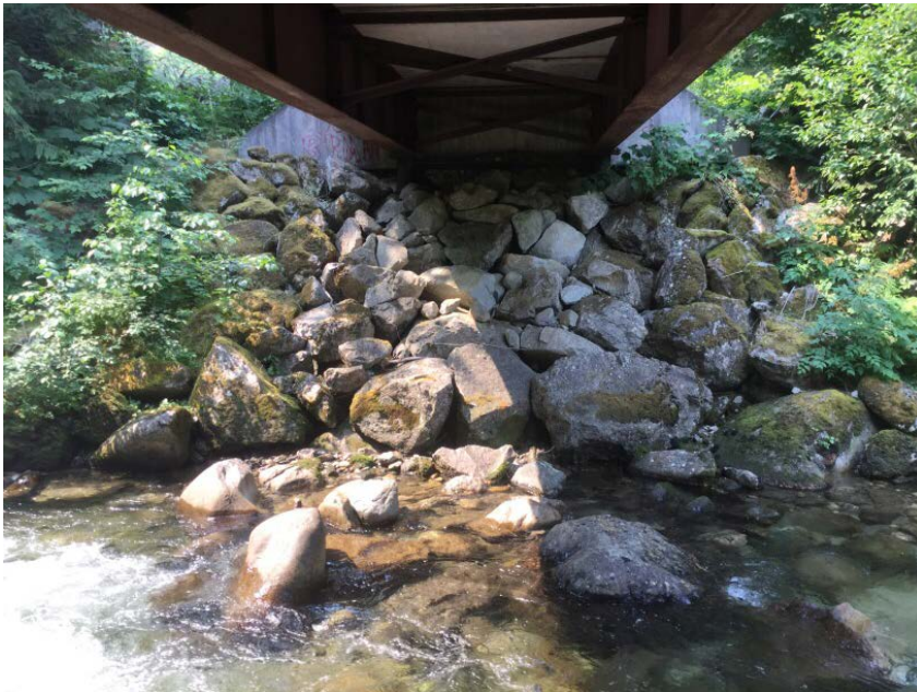
Left Bank Abutment when facing downstream
