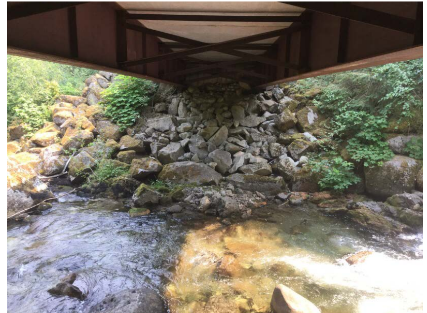
Right Bank Abutment when facing downstream
